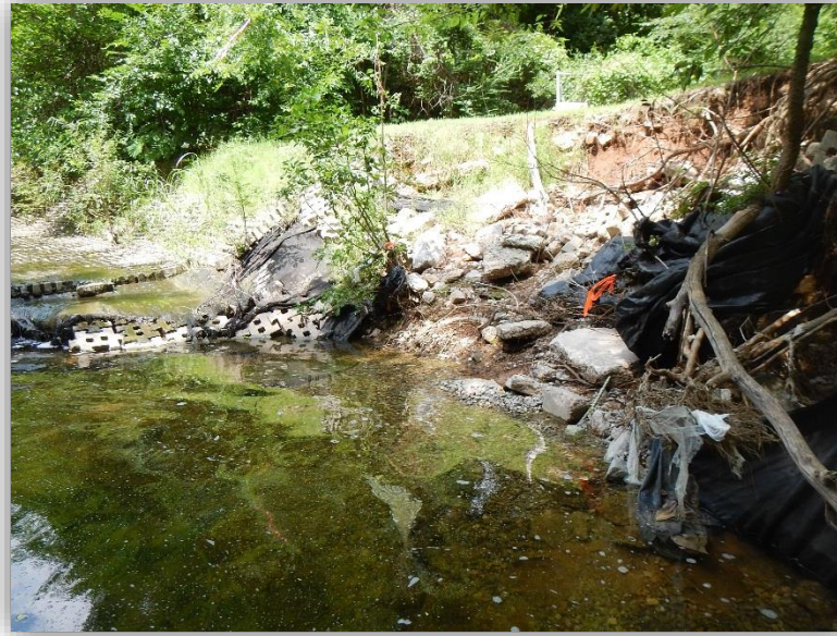
Figure 2: Articulated Block Channel Failure
