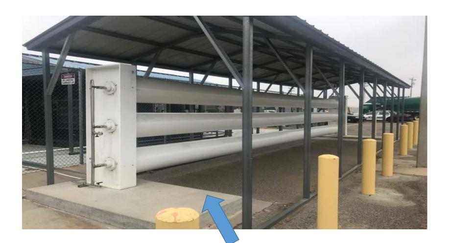
Space for an additional 3-pack CNG Storage Vessel
