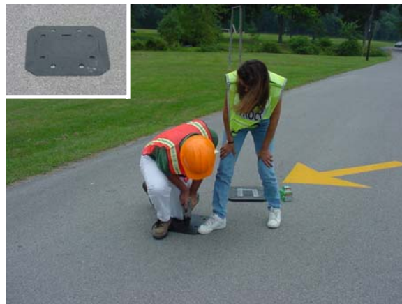
Figure 10-2 Electronic Vehicle Counter Installation (1)
