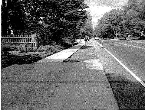
Bus Stop Pad and Sidewalk gap fill 700 Block W. Lindsey Street
