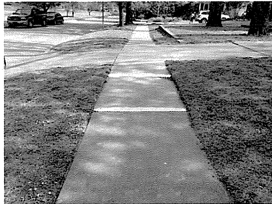
Bus Stop Pad and Sidewalk gap fill – 700 Block W. Lindsey Street
