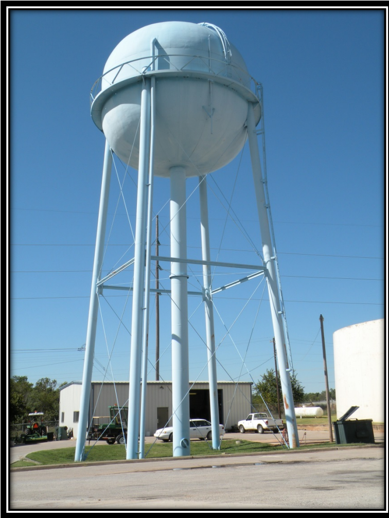
Water Treatment Plant Backwash Tower Last painted in 1993.
