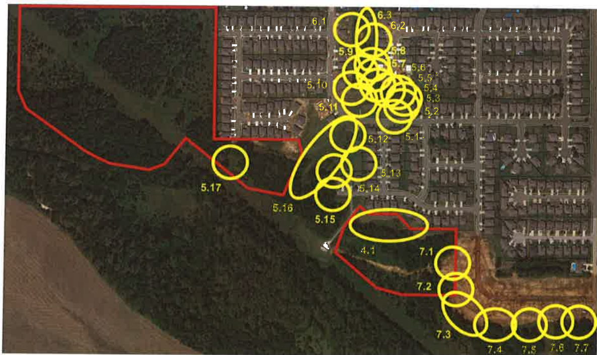
Figure 3: Major drainage/erosion issue areas (yellow circles). Photographs corresponding to each labeled region can be found on the following pages.
