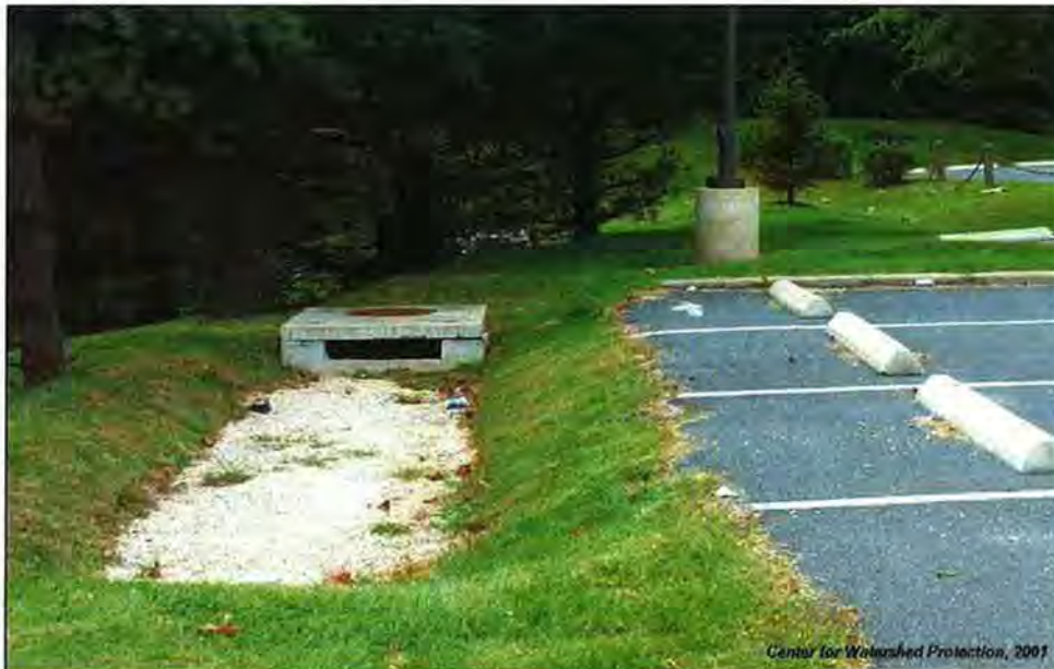
Figure 1: Infiltration Trench
