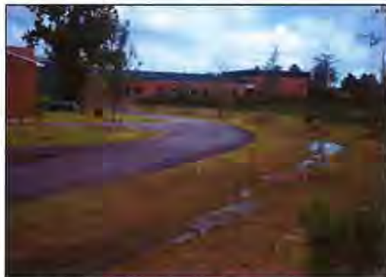
Figure 2: Wet Swale
