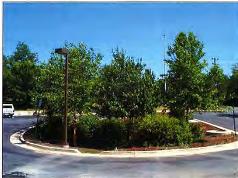
Figure 1: Bioretention created in a parking lot turn-around
