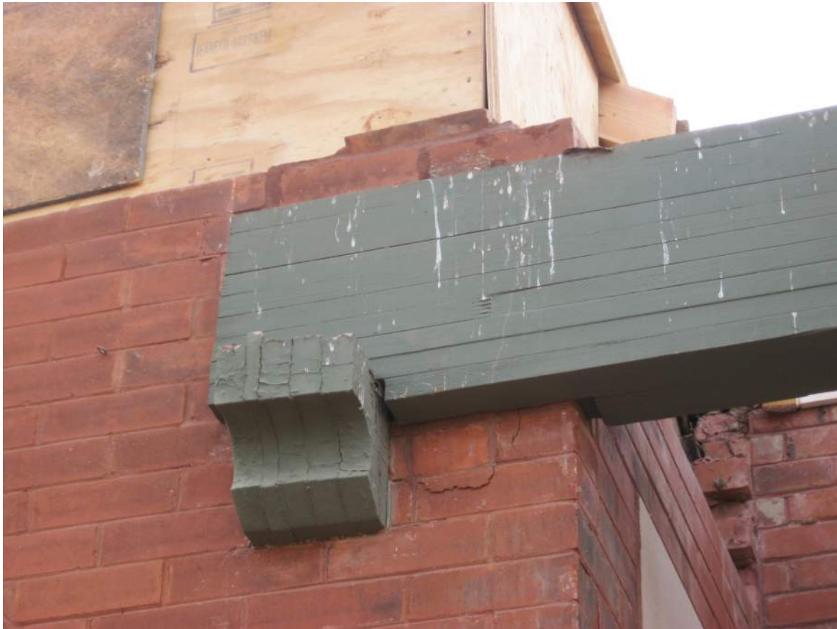
Photo 11 – December 2, 2016 – Roof Beam Support SW Corner below West Gable
