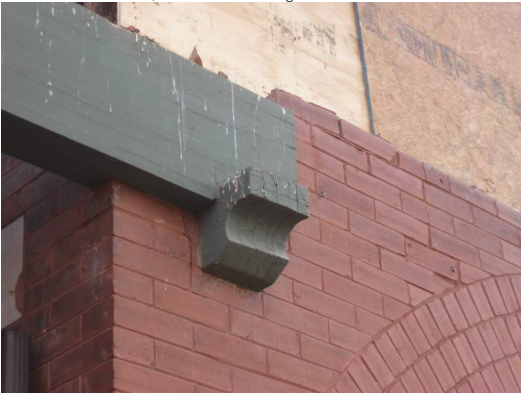
Photo 10 – December 2, 2016 – Roof Beam Support NW Corner below West Gable
