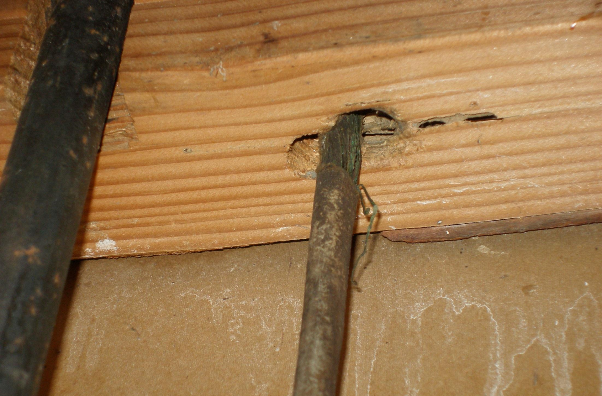
Damaged conductor sheathing leaves exposed wiring on this range circuit near the top of the wall.
