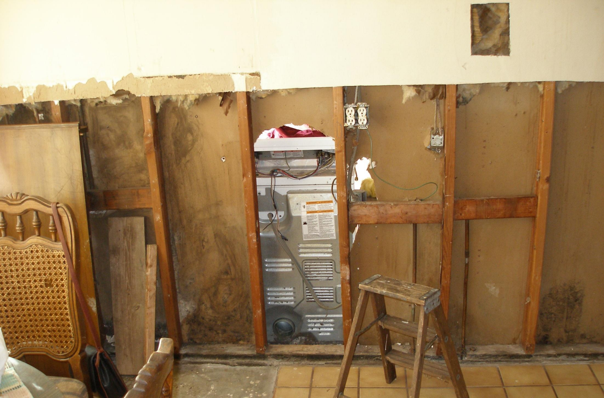
Looking from the kitchen into the garage where drywall is missing. This voids the required separation from the garage to the house.
