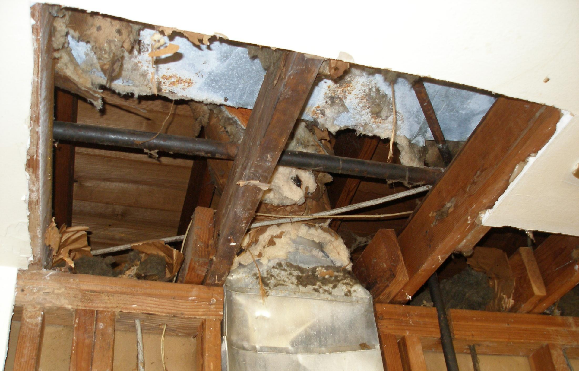
Kitchen ceiling above proper stove location. Lack of a ceiling challenges the ability to condition the air. Also difficult to maintain cleanliness and heightens the ability for fire or smoke to spread throughout the house.
