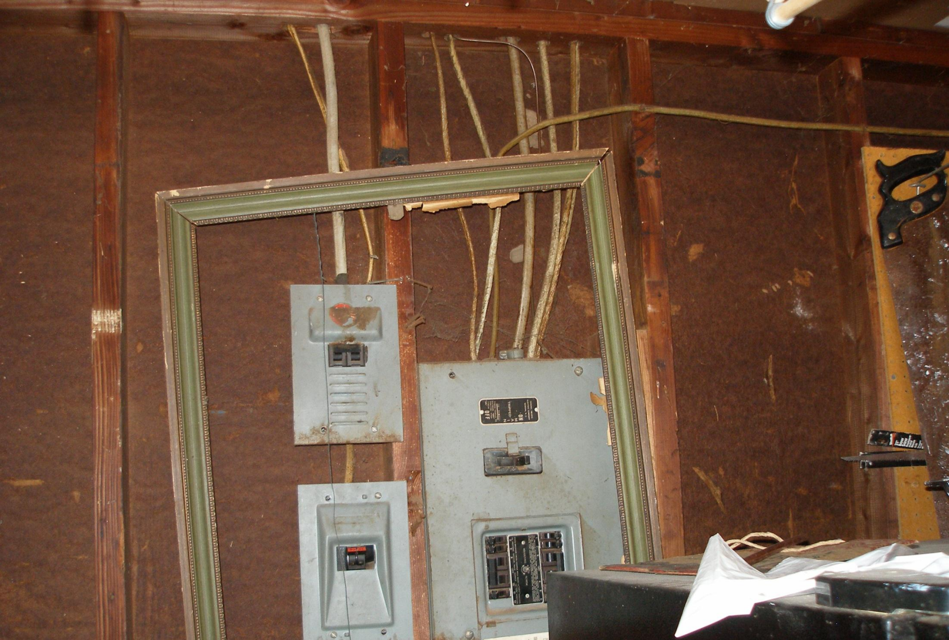
Electrical panels in garage. Drywall protecting panel wiring has been removed in the garage and in the kitchen.
