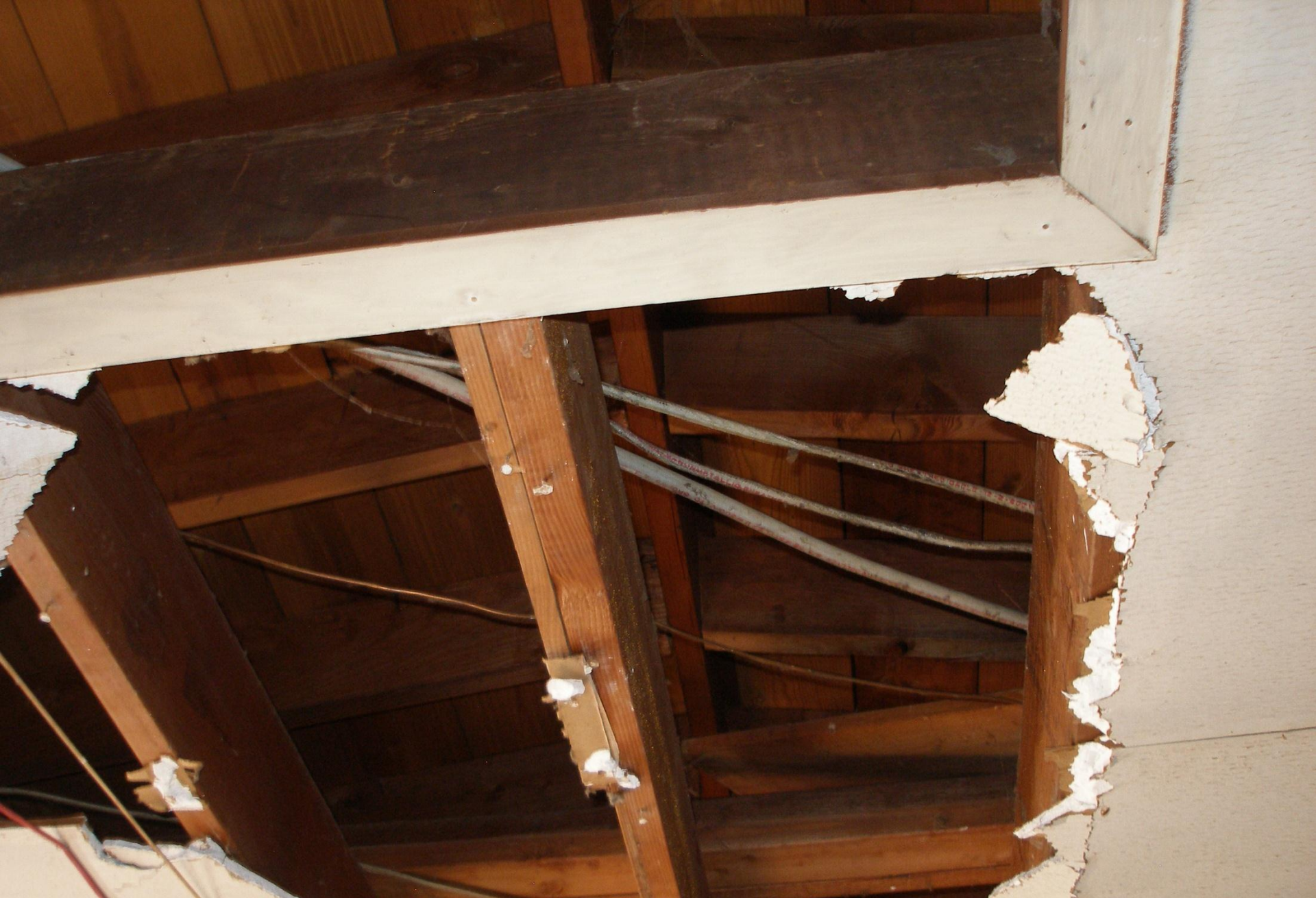
Missing ceiling in garage. The garage/house fire resistant separation is no longer intact.
