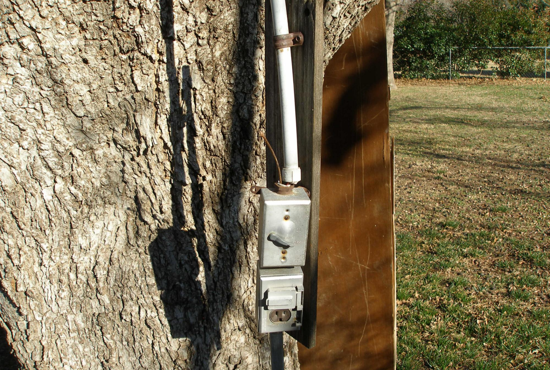
Broken conduit for exterior lighting with exposed wiring and open to allow water into box.
