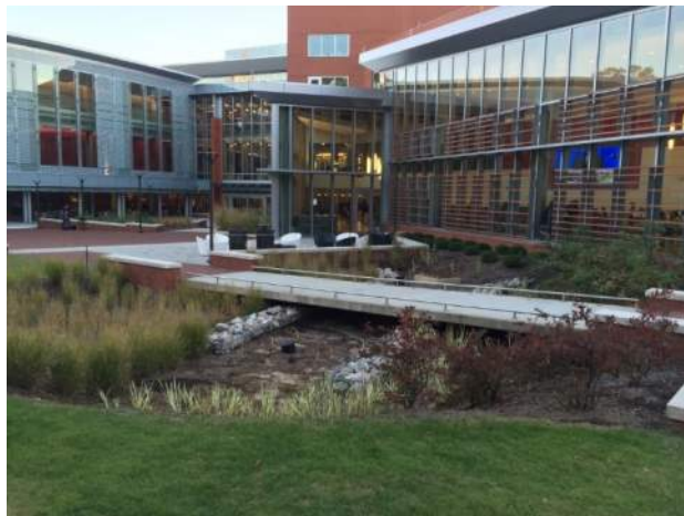
Bioretention / Rainwater Harvesting
