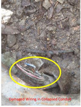
Intersection of Boyd Street and Classen Boulevard Damaged Traffic Signal Conduit, Pull Box and Wiring
