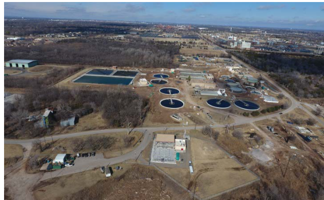
Water Reclamation Facility Expansion
