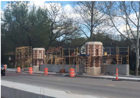
Lindsey Street Bridge over Imhoff Creek
