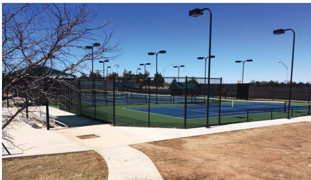
Westwood Tennis Center Improvements
