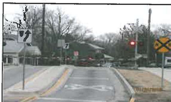
Automatic gates are provided for frequent crossings by BNSF's Mid-Con rail line
