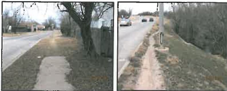
Examples of missing segments and well-worn paths are considered gaps within the existing sidewalk system
