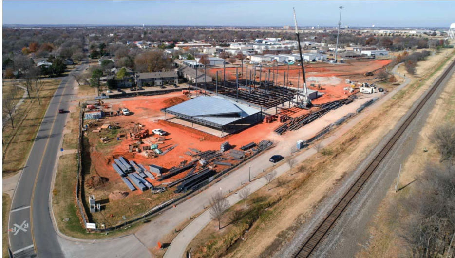
The new Norman Public Library, Central Branch
