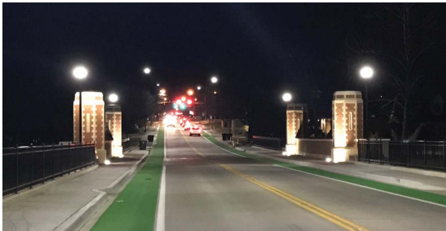
The new West Lindsey Bridge over Imhoff Creek
