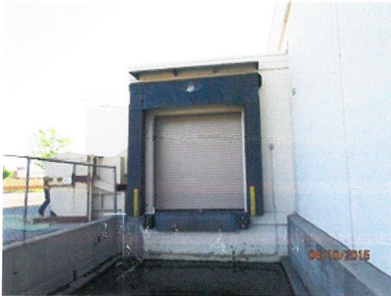
Document Name: loading dock.JPG
