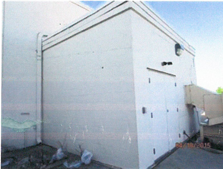
Document Name: no damage to south wall.JPG
