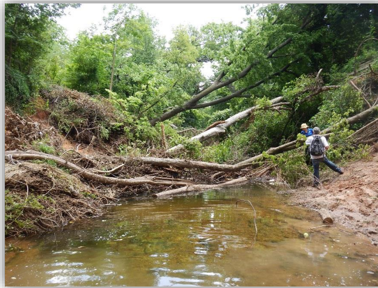
Figure 1: Stream Blockage - Vegetation
