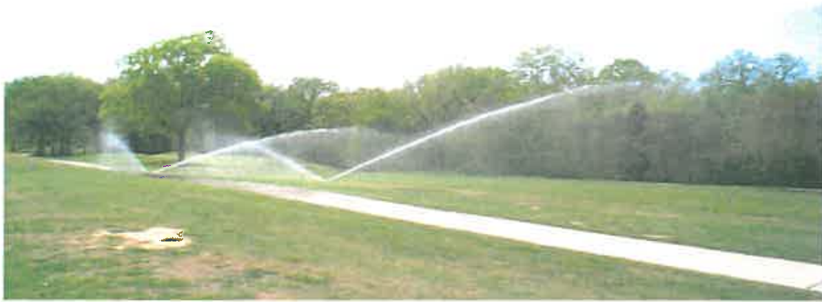
Figure 9 – City of Norman Treated Effluent Application
