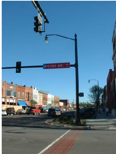
Stamped and Colored Intersections and Cross Walk Edges
