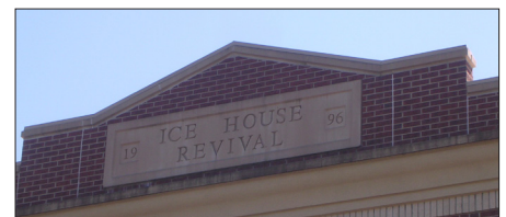
Masonry parapet sign
