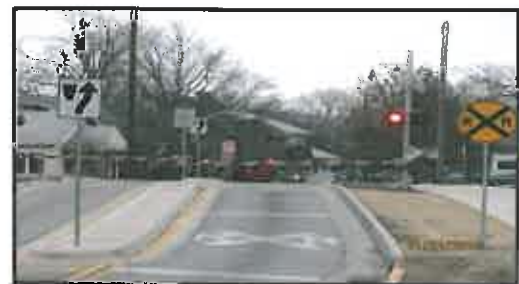
Automatic gates are provided for frequent crossings by BNSF's Mid-Con rail line
